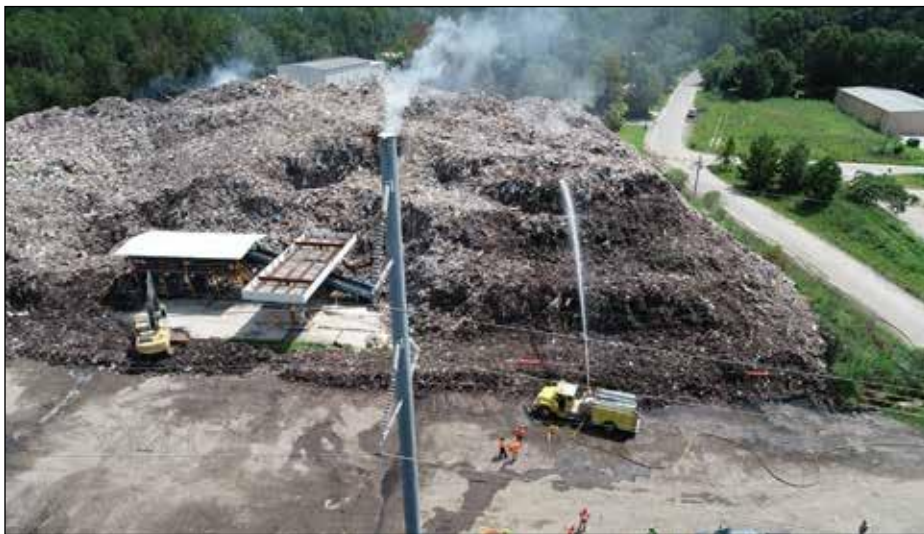
Pictured left is an aerial view of the Able Contracting Site showing a pumper truck spraying water on a hot spot in August 2019.
