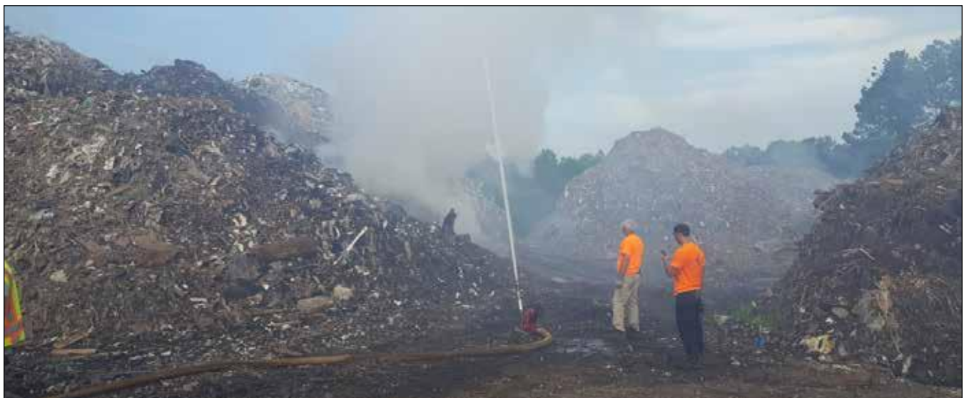
Firefighters reposition a ground-based water cannon to a hot spot at the Able Contracting Site.
